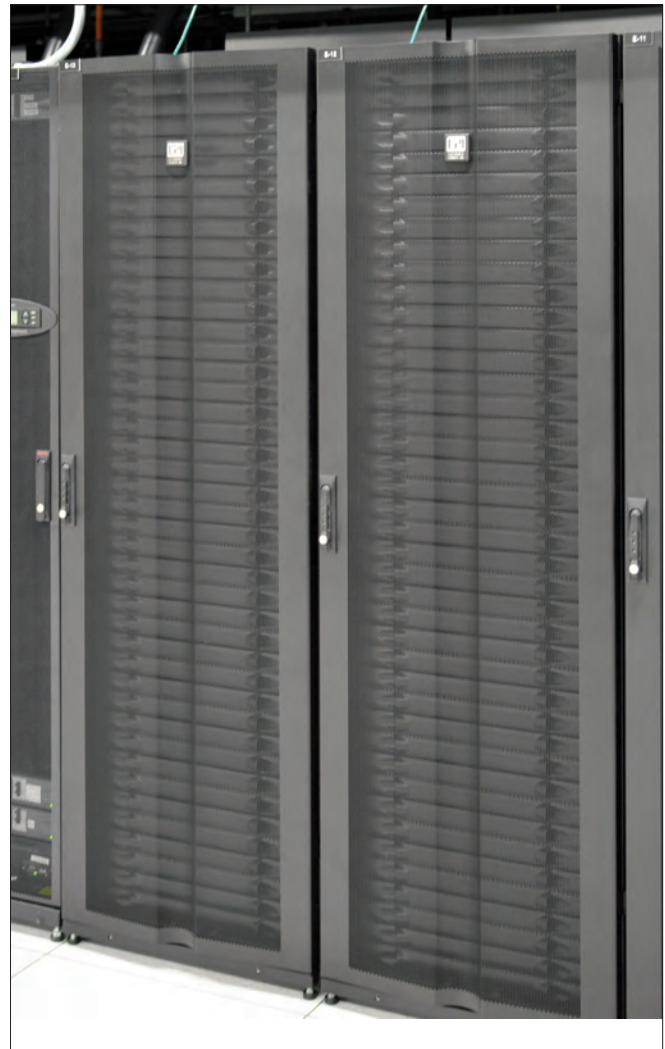
CPI's GF-Series GlobalFrame Cabinets with custom doors, support baffles and Hotlok® Snap-In Filler Panels were installed to improve airflow efficiency in Cologix's Dallas data center.
